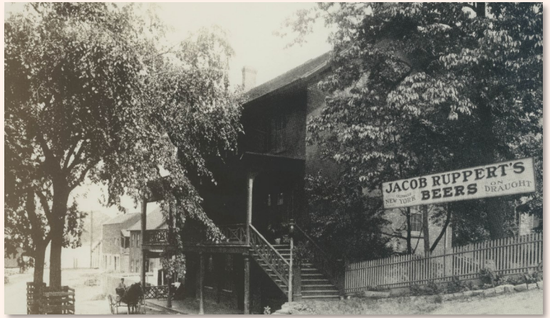
Dock/Ferry House & Golden Eagle Hotel/Garrison Hotel, c. 1892.
